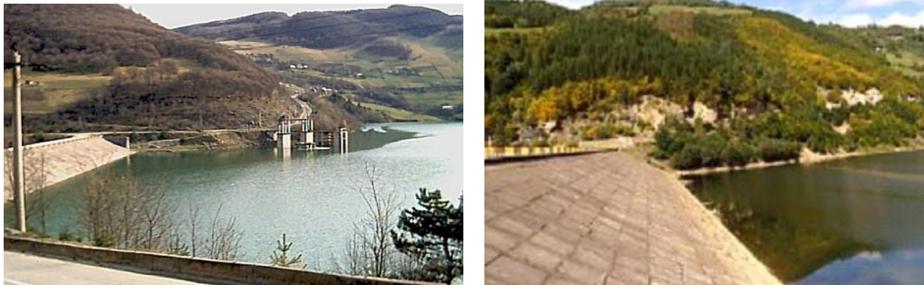
Figure 2- General view of the Mihoiesti Dam.
