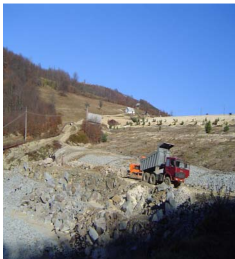
Figure 3- Valea Săliștei tailing dam –lower benches, with leveling and ballasting operations.
