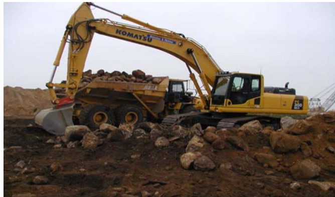
Figure 11: Hydraulic excavator to extract stones and rocks
