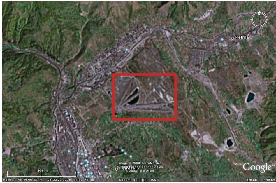
Figure 2. The five branches structure of waste dump Petrila
