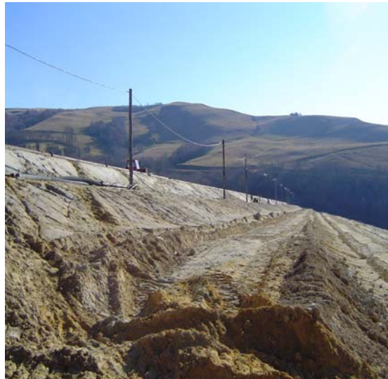
Figure 2- Valea Săliștei tailing dam –elevation talus, upper benches.
