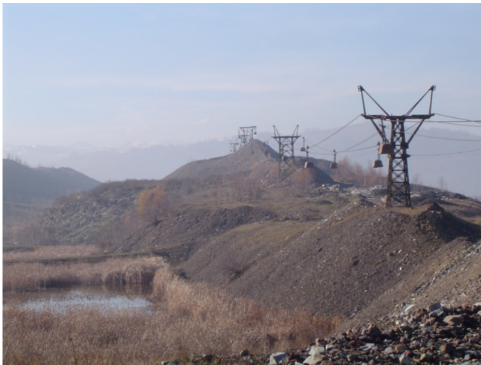
Figure 3. The aerial ropeway transport system
